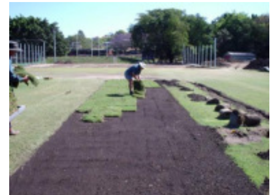
Figure 6: - Laying full turf on new wicket.
