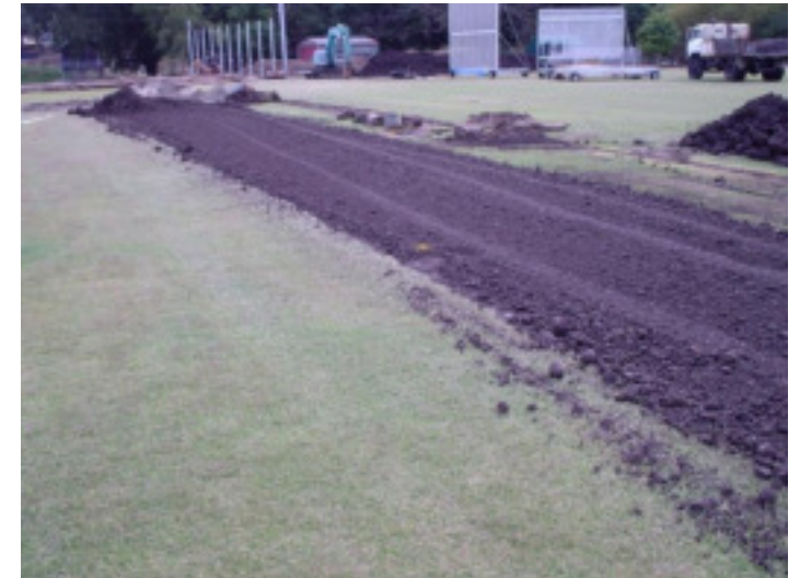
Figure 14 - Spreading of black soil
