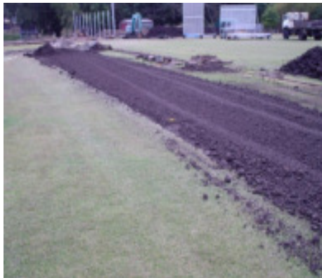
Figure 1: Spreading and levelling wicket soil
