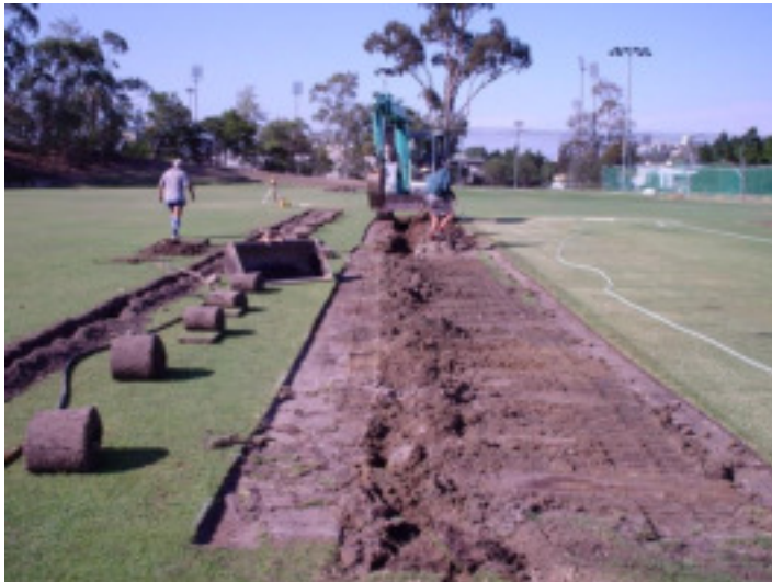
Figure 15 - Excavating wicket site
