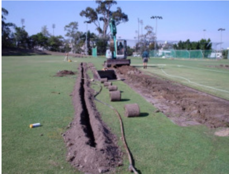
Figure 17: - Irrigation line 3m from Wicket Block
